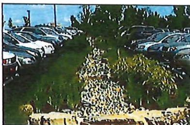
Parking Lot Island dual functioning to infiltrate stormwater
