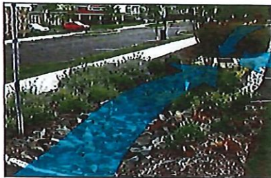
Bioswale "cleansing" stormwater before infiltration
